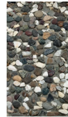
Wasch Concrete Facing Work
